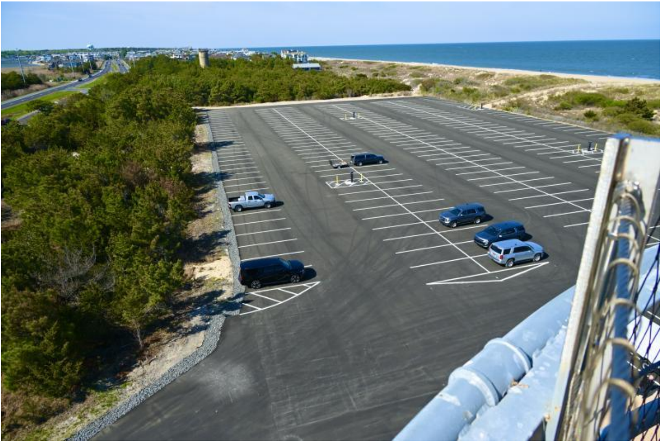
The Delaware Seashore State Park bathhouse has a new parking lot and handicapped-accessible ramp.
