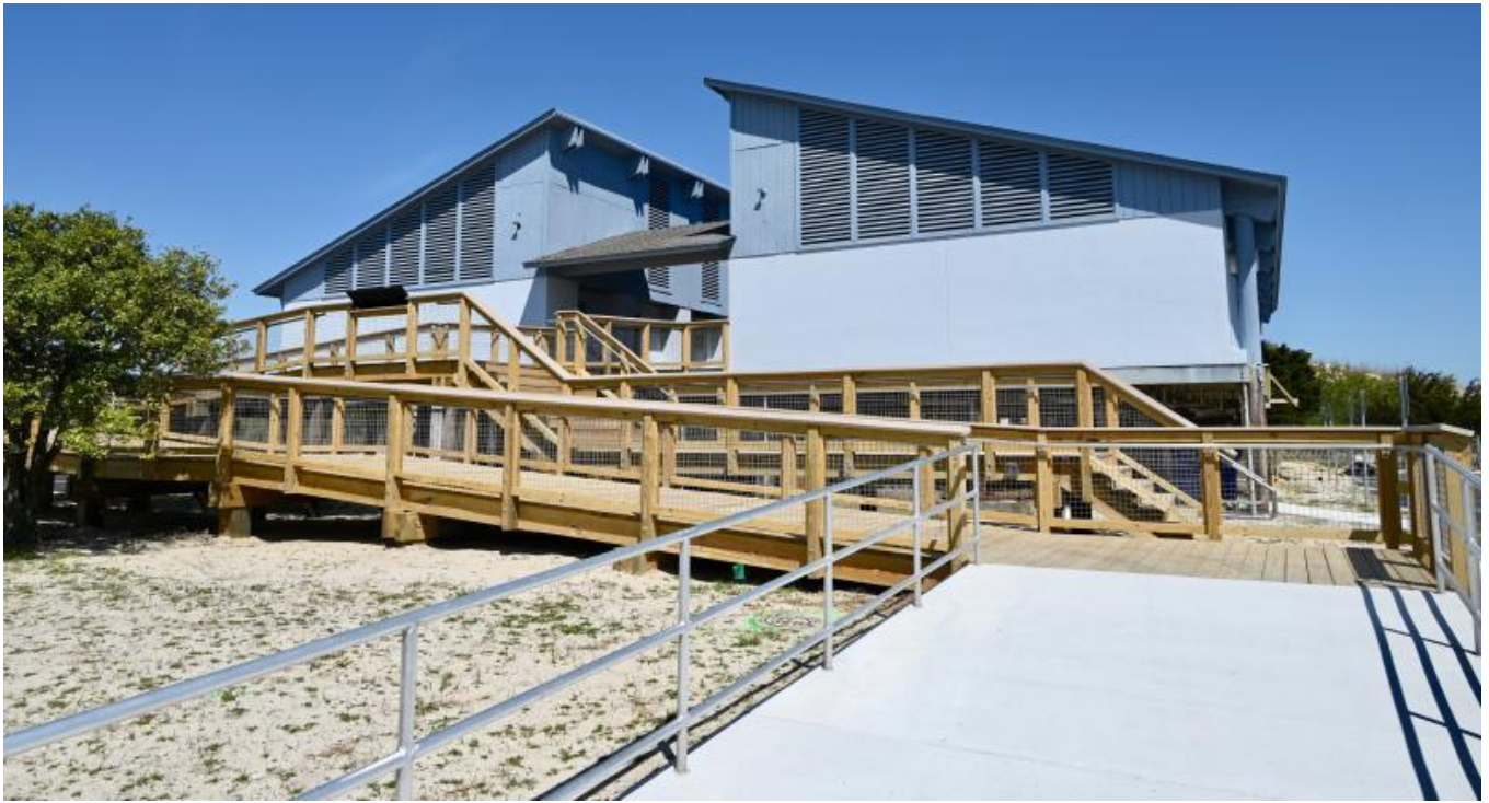
The Towers Beach bathhouse has a new handicapped-accessible ramp, as well as a new parking lot.
